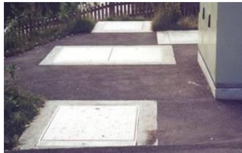
Manhole covers SD 8: back-up proof, load-bearing
