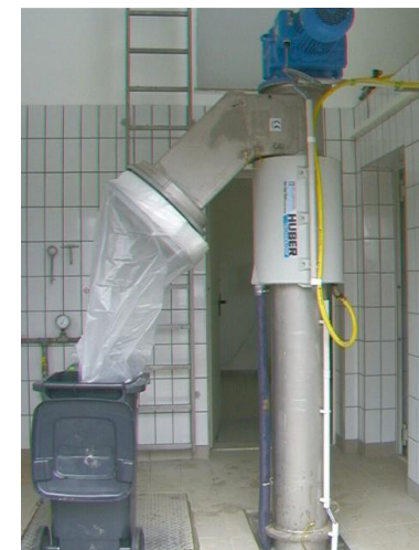
RoK 4 Screen for Baar pumping station (Germany)
