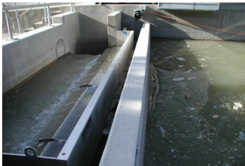
ROTAMAT® Storm Screen for stormwater discharges RoK 2 at an overflow
