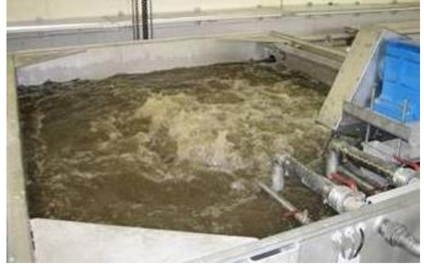
Filtration tank, HUBER BioMem@ plant
