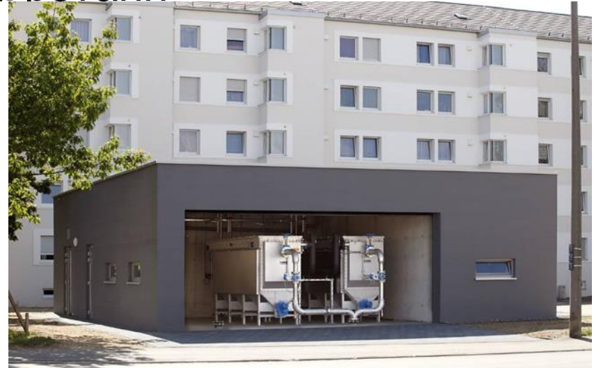
HUBER Heat Exchanger RoWin installed in a building
