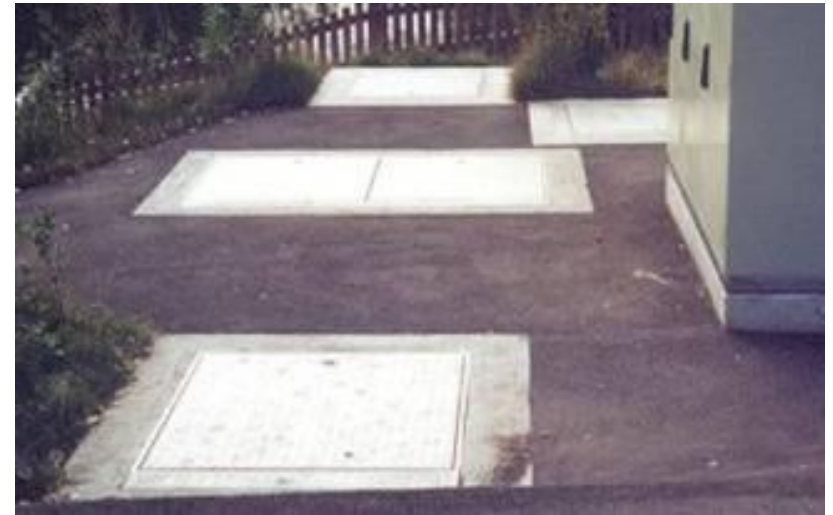
Manhole covers SD 8: back-up proof, load-bearing
