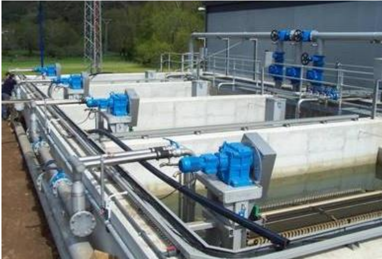
4 VRM@ 30/448-Units in filtration chambers
