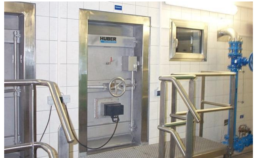
Pressure door TT 7 with central lock and spotlight
