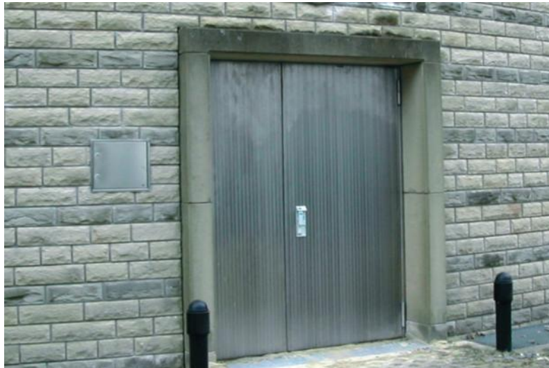
Double-wing safety door TT2.2 / WK3
