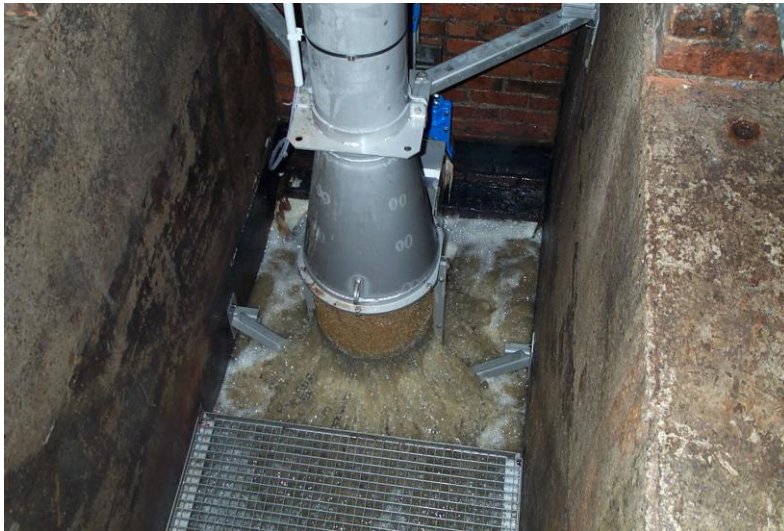
HUBER Pumping Station Screen ROTAMAT® RoK4
