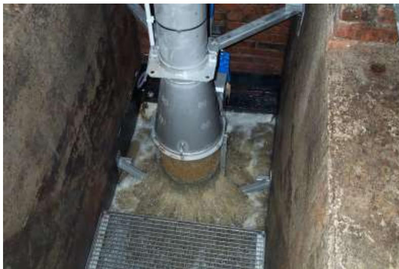
HUBER Pumping Station Screen ROTAMAT® RoK4
