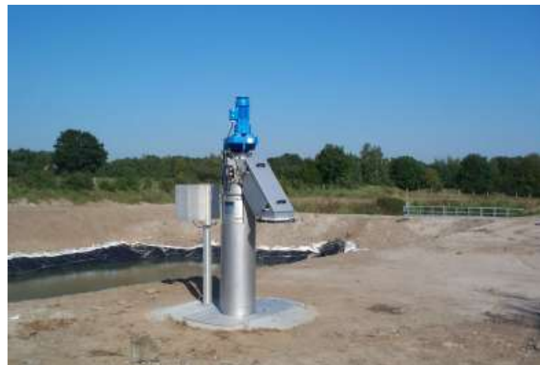
HUBER Pumping Station Screen ROTAMAT® RoK4
