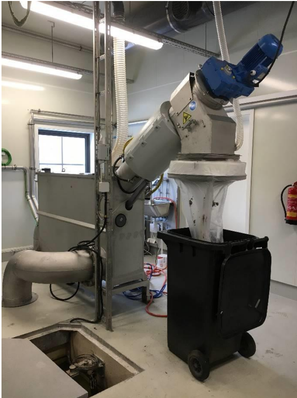
Ro9 i tank
