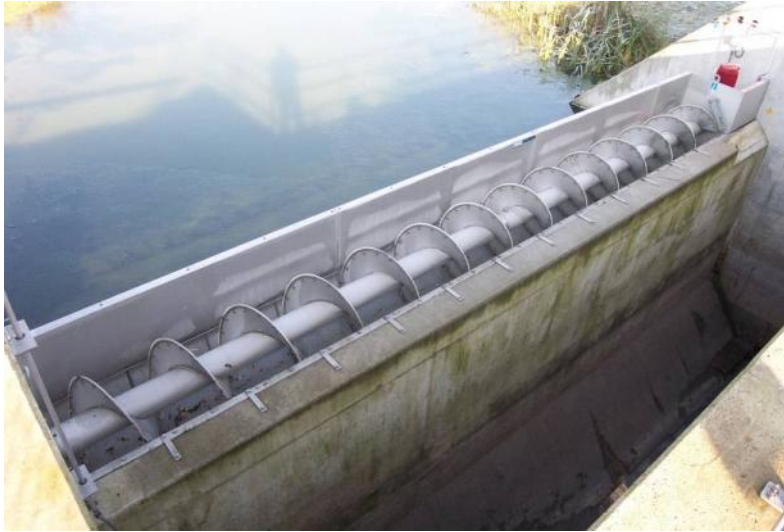
HUBER Storm Screen ROTAMAT® RoK1 at an overflow discharge
